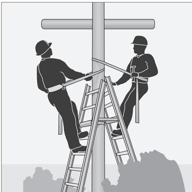
Figure 15 Pole straps used with portable ladders.
